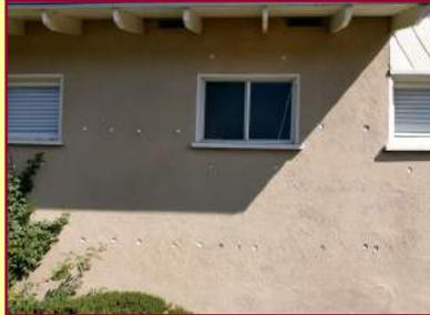
~ The rental house was built with no air-conditioning and no insulation. A couple of summers ago, we had full air-conditioning installed, and just recently we added insulation to the attic and the south and west walls. You can see the holes, through which the insulation was added. Pete Tuzzolino will be repairing and painting the wall within the next couple of weeks.
